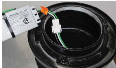
STEP 2: CONNECT WIRES IN CAPITAL TO DRIVER ASSEMBLY
