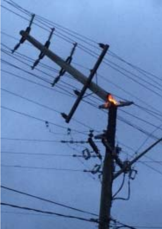
A [wood] pole fire causes a power outage that affects 30 000 PowerStream customers March 2015 for several hours.
